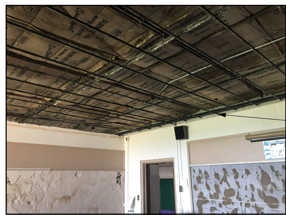
E1 TYPICAL CEILING SUPPORT/FRAMING SYSTEM NTS
